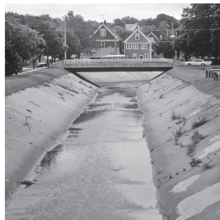
Note the presence of any artificial embankments. This stream has a fortified concrete embankment.
